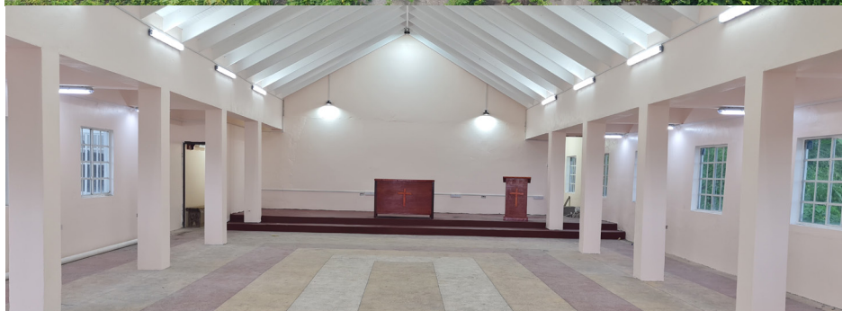
“After” images of repairs done to the Church structure
